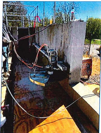
Work completed to drain and clean, sawcut, inspect and repair existing Chlorine Contact Channel for new UV system.
