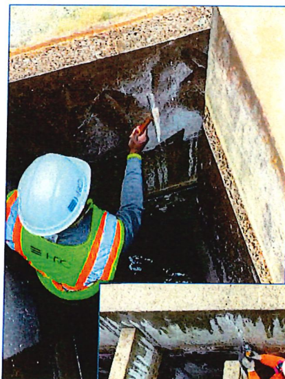
May 7 th Groundbreaking and grading and concrete removal at Chlorine Contact Tank for New UV System and Building.
